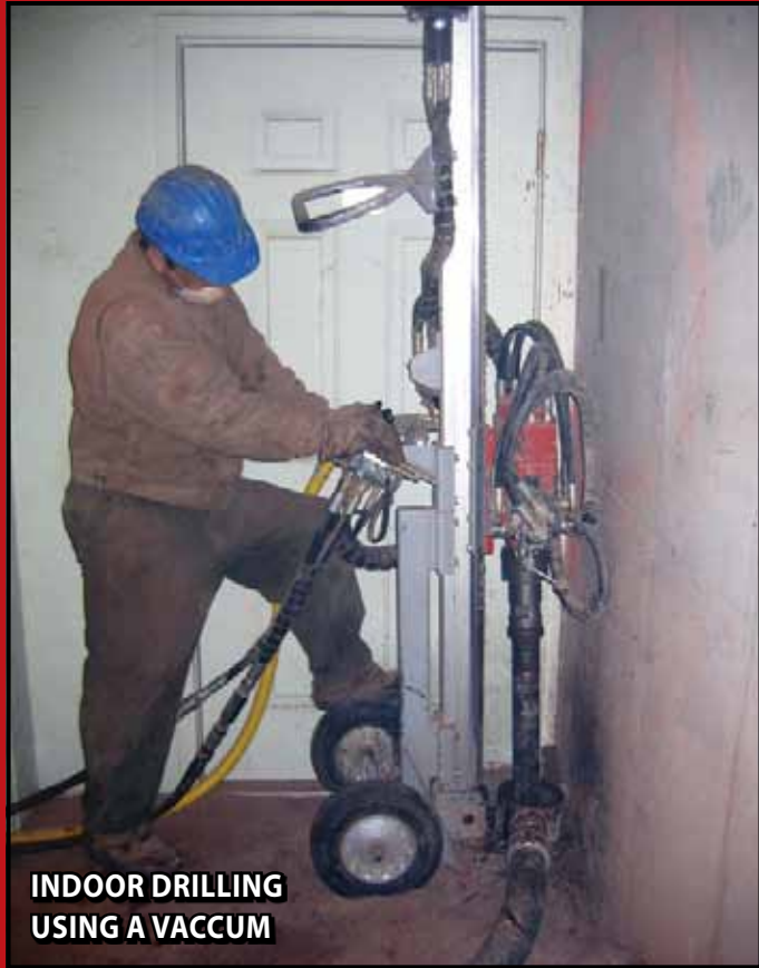
PRE-DRILLING FOR RESISTANCE PIERS
