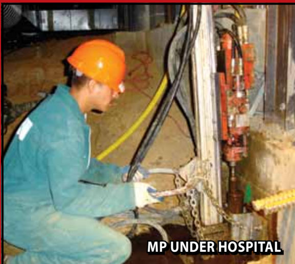
JACK USED FOR RESIDENTIAL FOUNDATIONS
